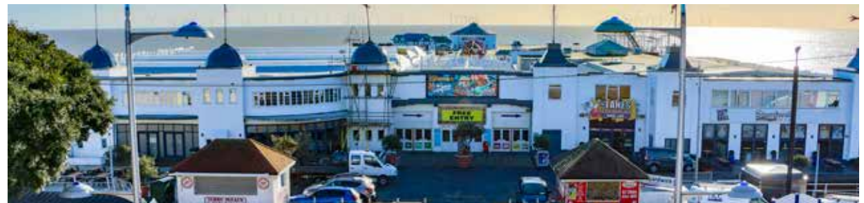
Figure 17 View of Clacton Pier
