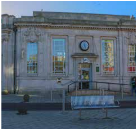
Figure 24 Lloyds Bank Building
