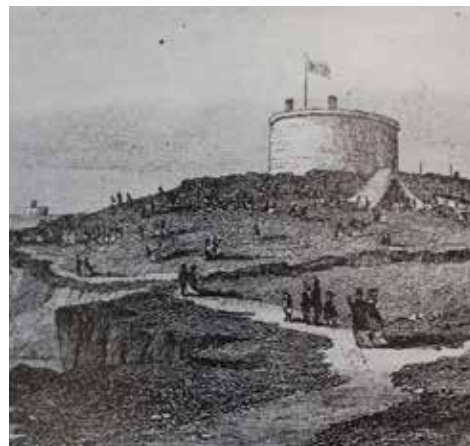
Figure 3 Martello Tower F 1880 (Britain in Old Photographs 1995)
