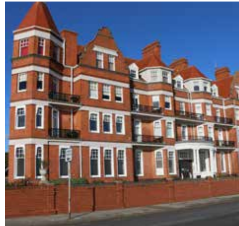
Figure 34 Colchester Institute (Grade II Listed)
