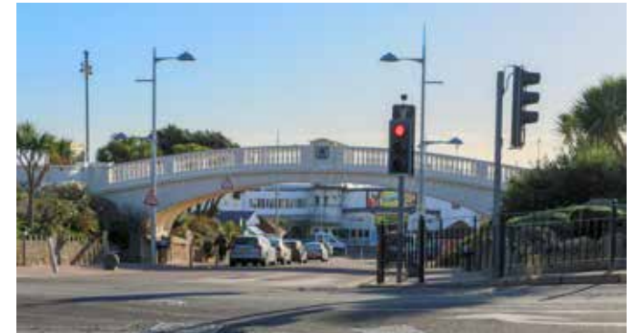
Figure 21 Pier Gap Bridge (looking South)
