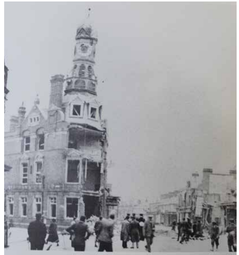
Figure 12 Air Raid Damage 1941 (Britain in Old Photographs 1995)
