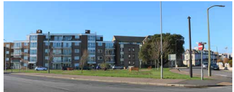
Figure 53 Development on the west side of Anglefield Junction
