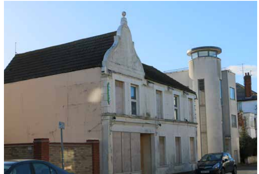
Figure 52 Vacant property on Rosemary Road
